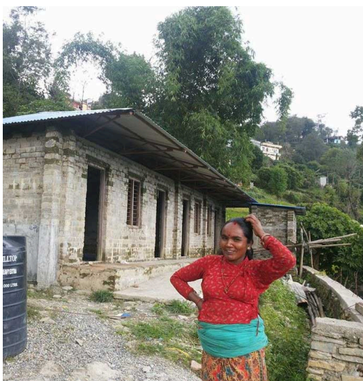
...to this. The first Guy Joseph ECDC is almost finished!
